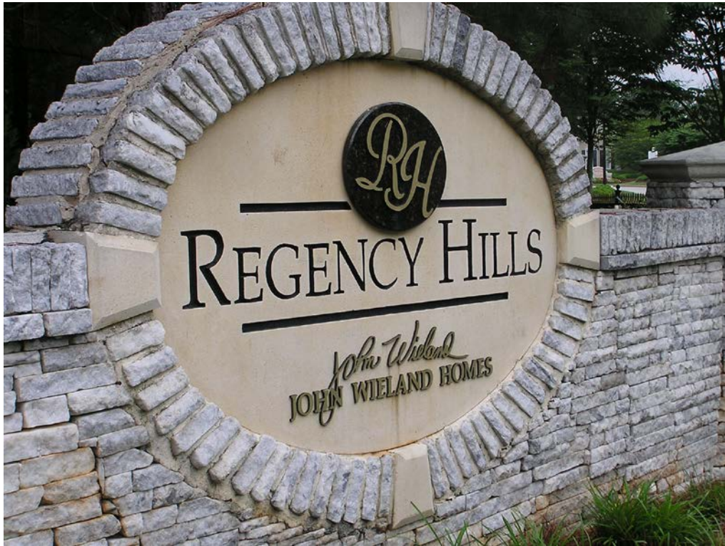
3. View showing the stained and dirty logo sign at the property entry.
